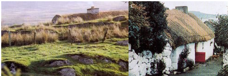
Figure 7 and 8: These are examples of single-storey houses of modest sizes, usually containing one room. The plan was rectangular with walls made from local stone with thatched roofs. These dwellings blended easily into the Irish landscape due to the use of local materials.
