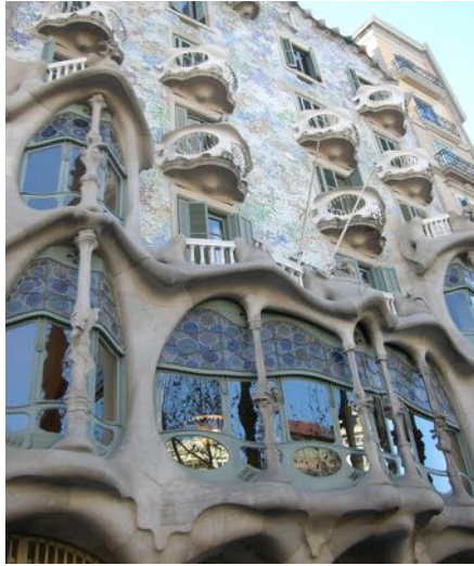
Figure 3.10 Casa Milà Facade
