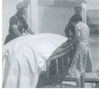
Right: Putting canvas on a currach 1940. Currachs today are made from a laths structure, canvas and tar.
