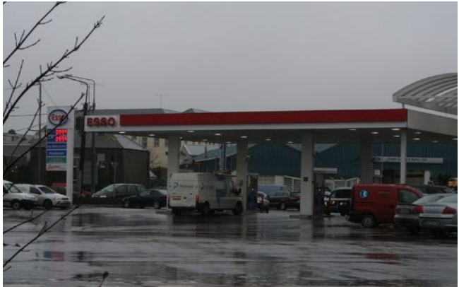
7- Typical Station today
