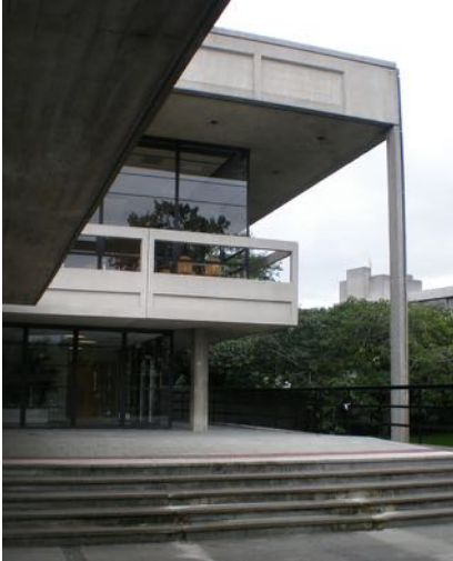
Robin Walker's Restaurant Building
