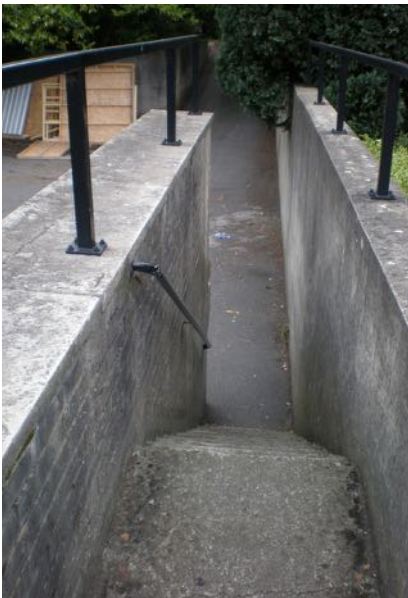
Restaurant Building Staircase
